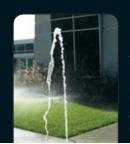
At 40 psi, the standard pressure fixed spray with a missing nozzle wastes water at a rate of 40 GPM.
